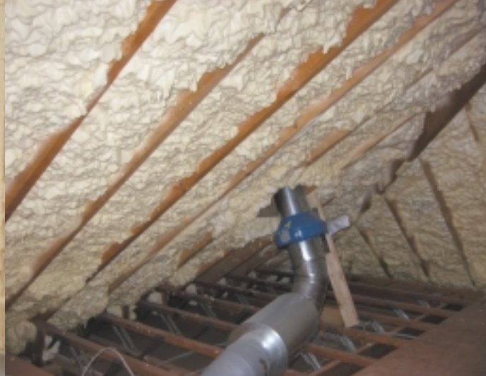
Attics and Ceilings
